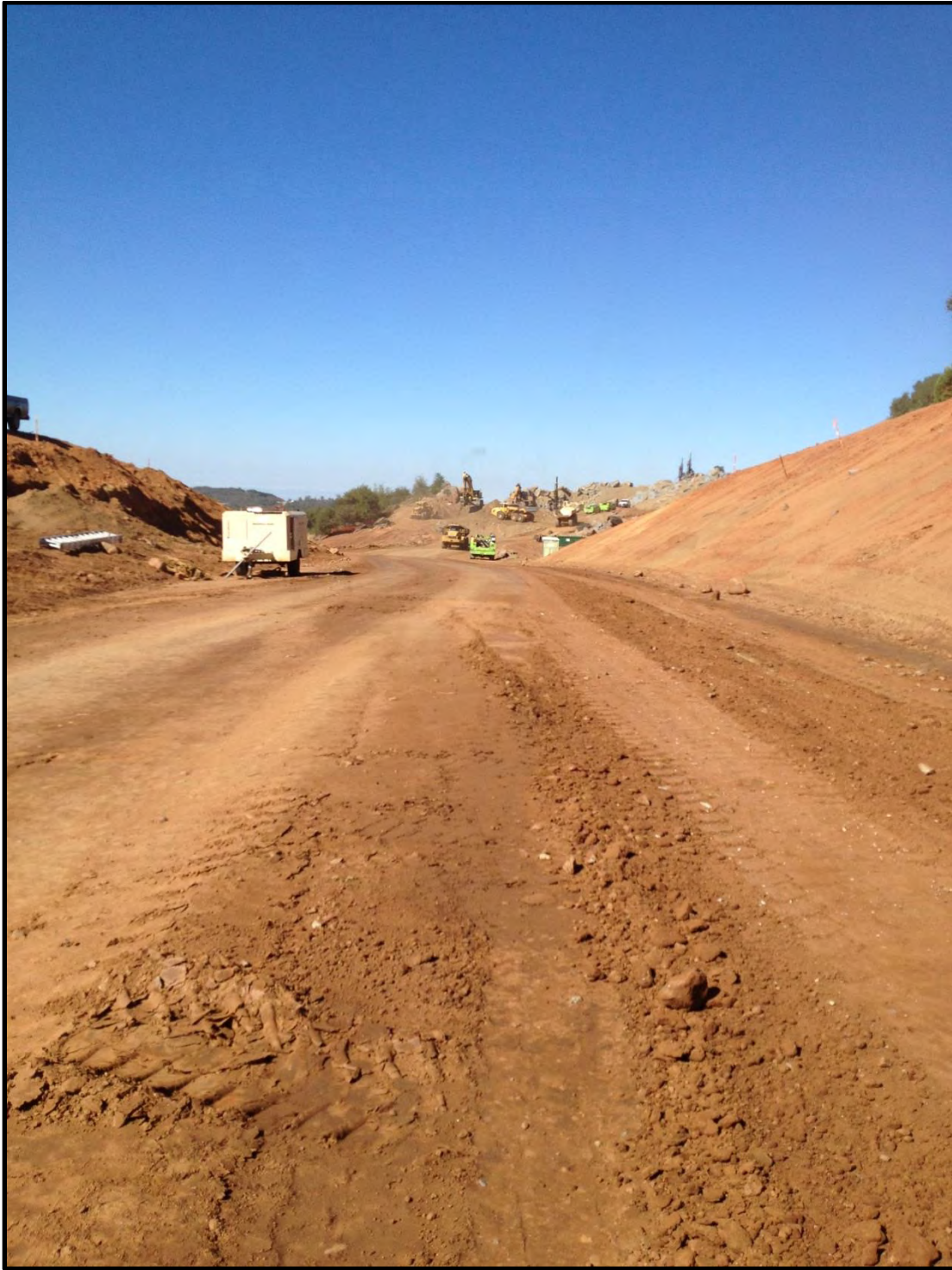
Figure 3.1 Construction on East Sonora Bypass Phase II – 2013, Photo Courtesy of TCTC
