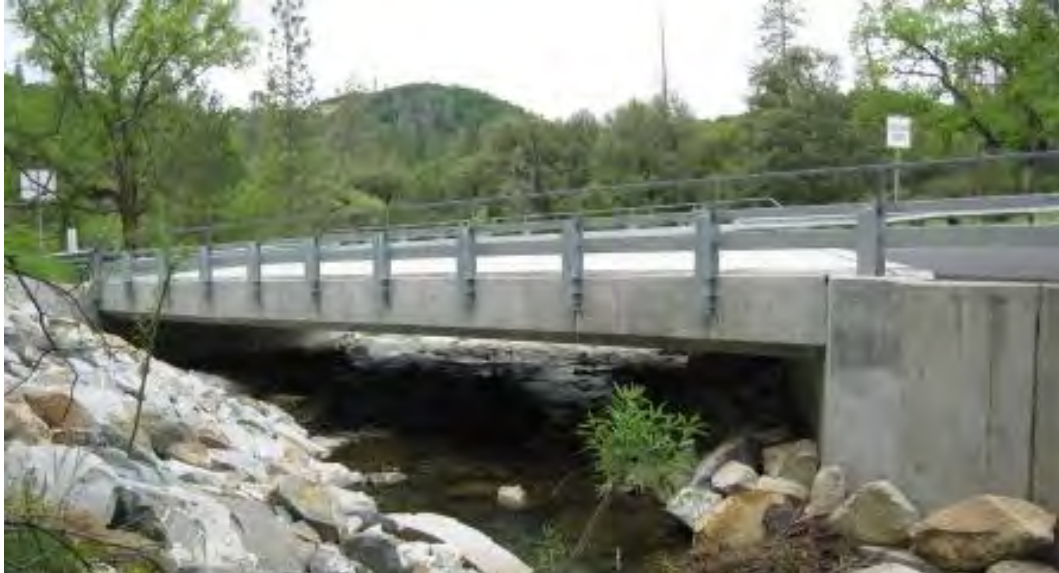
Figure 6.4 Phoenix Lake Rd Bridge Crossing Sullivan Creek
