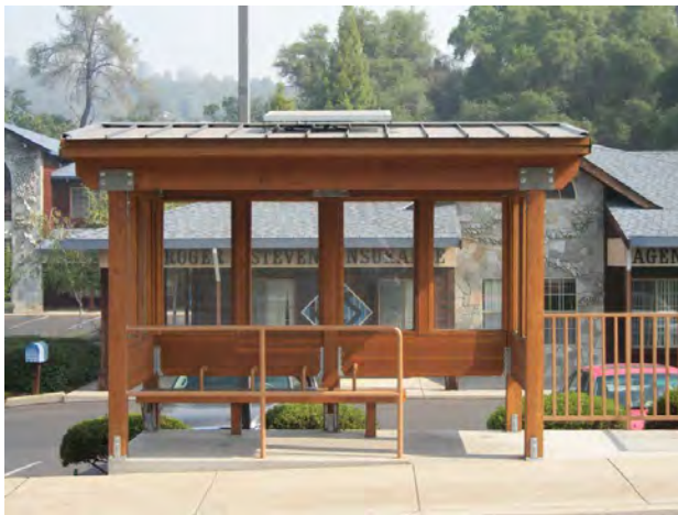
Figure 10.2: Indian Rock Bus Stop along Mono Way
