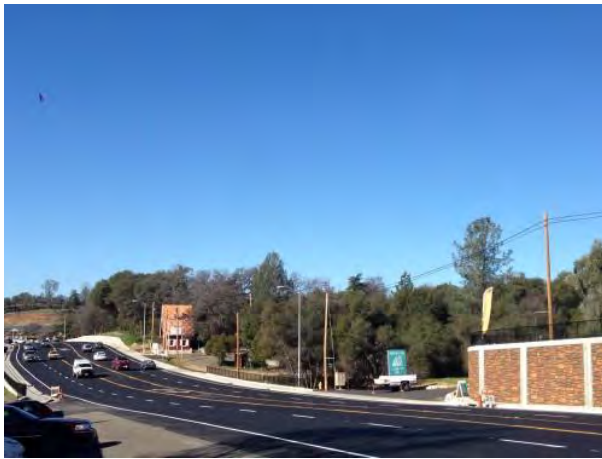
Figure 6.2 Mono Way Widening Project
