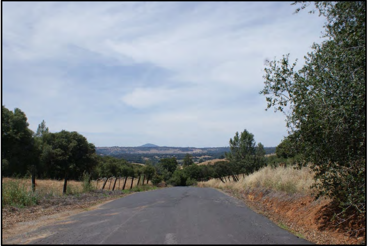
Figure 6.1 – Algerine Road in Tuolumne County – Photo Courtesy of TCTC
