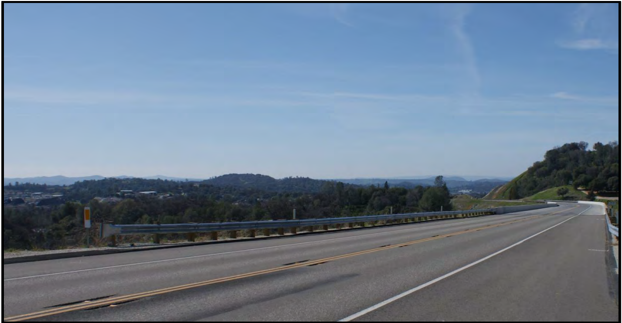
Figure 5.2 - East Sonora Bypass Stage II
