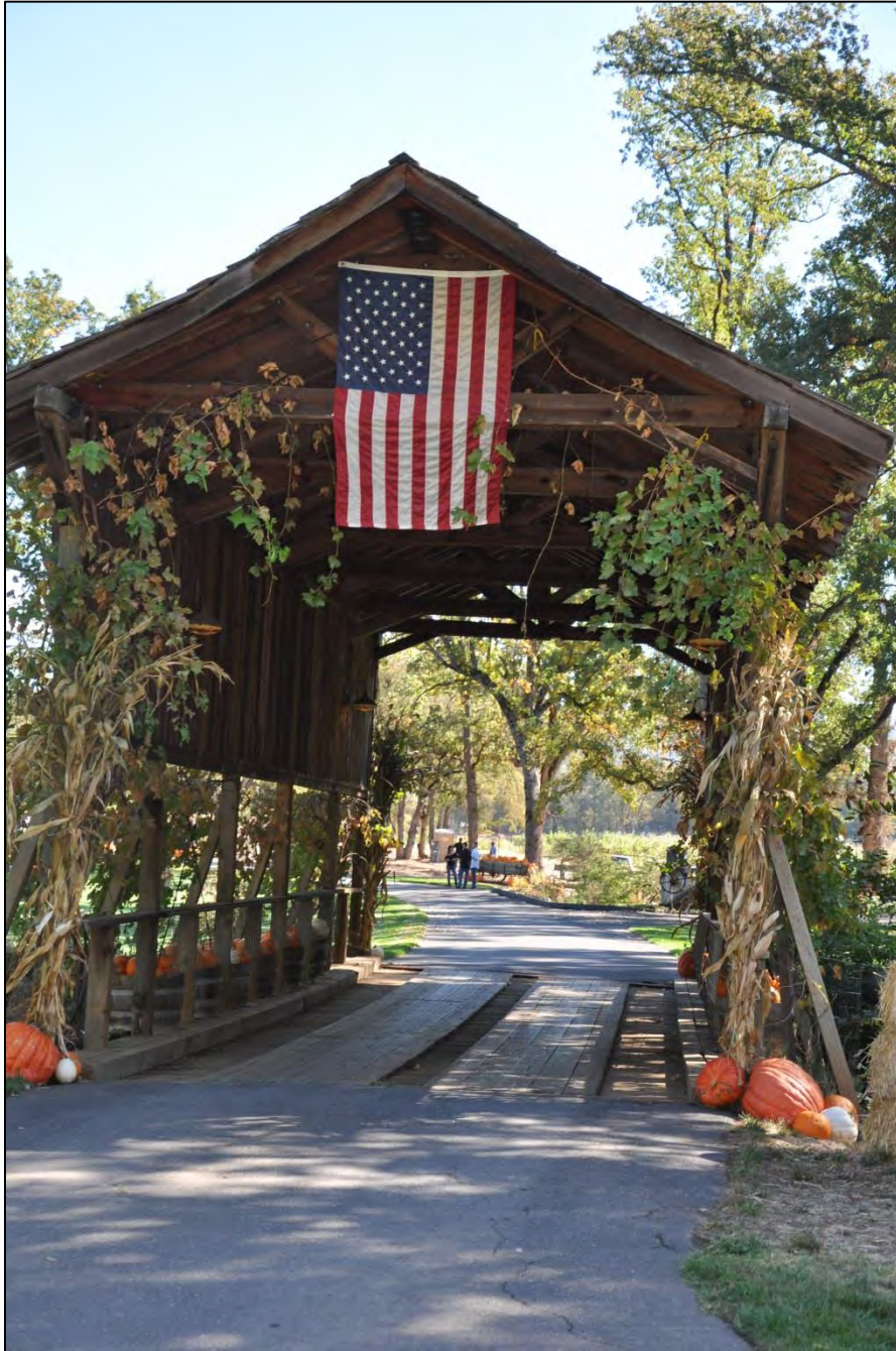
Figure 2.1: Covered Bridge, Photo Courtesy of Tuolumne County Visitors Bureau
